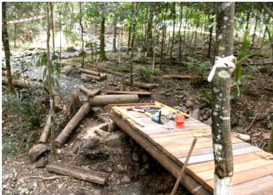
Construction of footbridge over Grandis Creek nearing completion
